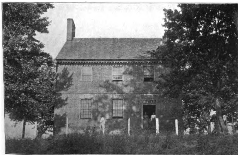
LEE MANSION (COLONIAL), NORTH WEST FORK RIVER.
